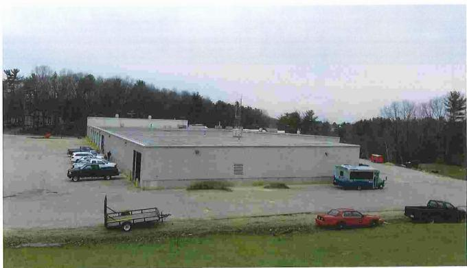
Public Works and Fire station roofing (roofing in the forefront is in very bad condition) Roof top heating and cooling systems for the offices and fire department located on back roofing area
