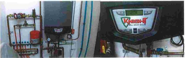
Radiant Boiler and piping (excellent condition)
