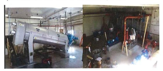
The picture above on the left is the new Huber screw press that will dewater the wasted solids from the treatment process. The solids will be thickened from approximately 1% solids to 24% solids. The above right picture is of the new pumps and process piping in the control building.
