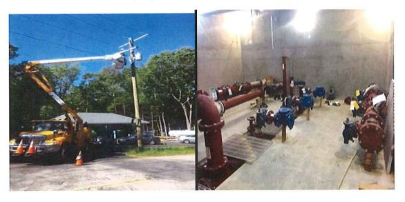
The above picture are of PSNH installing the transformers at the Blending Facility, and the process piping in the basement of the facility.
