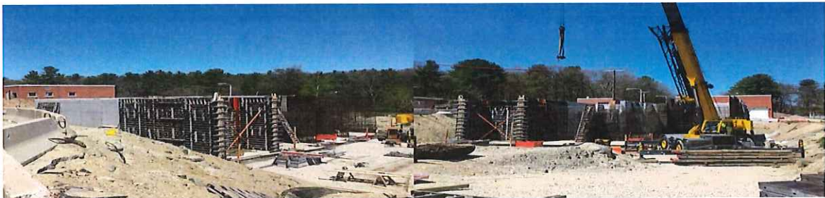
Aeration Walls formed for concrete
