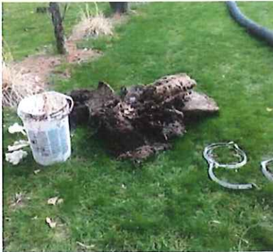
Roots Pulled Out of Manhole
