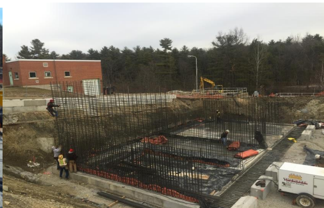
Aeration Basin Wall Construction
