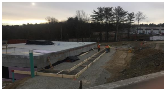
Frost Wall for Control Building Slab
