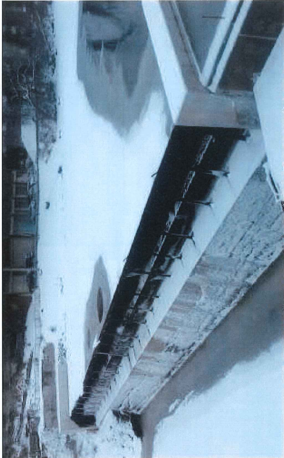
Obermeyer Spillway Gate system. Jackson Falls Dam, Nashua, NH Image Source: GZA Phase I Inspection
