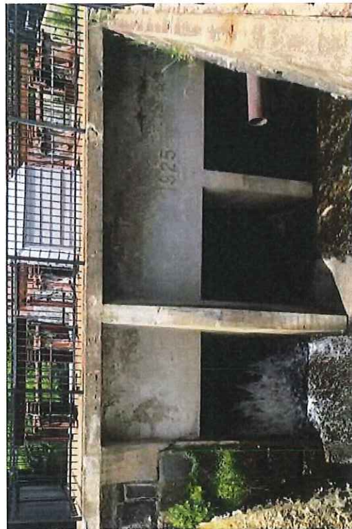
Leakage at gate structure
