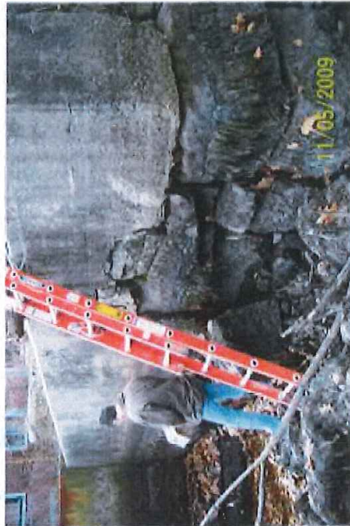
Photo A, Crack behind ladder
