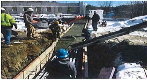
Electrical Duct Bank for the Control Building
