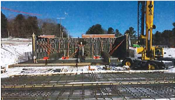
Aeration Walls formed for concrete
