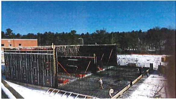
Aeration Basin Wall Construction
