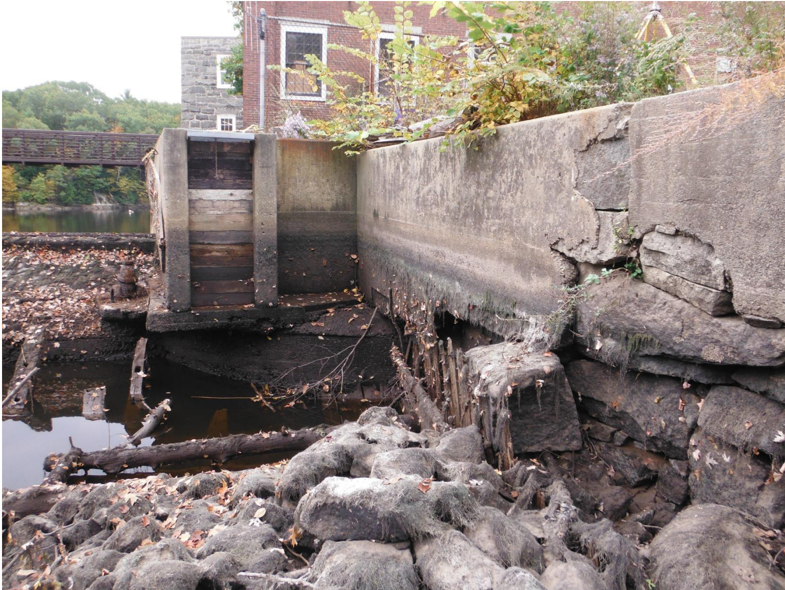
Figure E-4: View of the dam's right abutment, fish ladder and a portion of the legacy timber crib dam. Photograph taken 10/4/2013.
