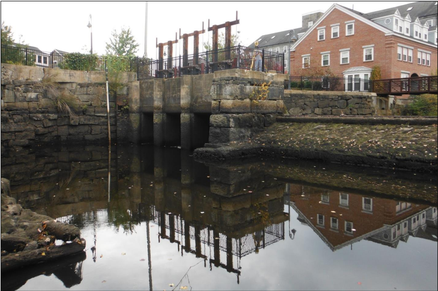
Figure 2.2-3: Left abutment and crest gates. Photo taken during the October 2013 drawdown.
