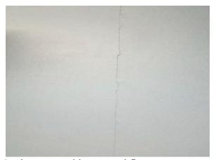
Settlement cracking second floor access
