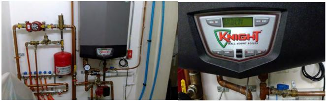
Radiant Boiler and piping (excellent condition)
