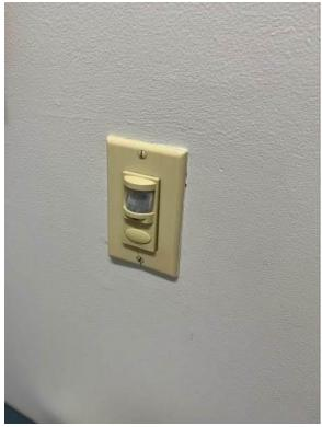
Lighting control for most spaces(line voltage occupancy sensors)
