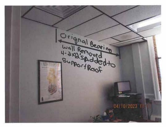
Third floor portion of bearing wall removed. New partition wall terminates at ceiling grid
