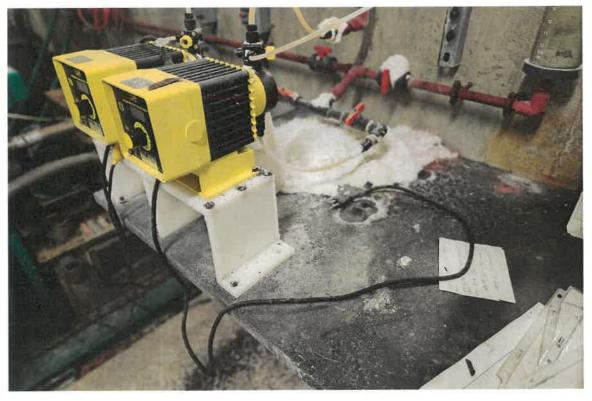
Pump and pipes in the chemical storage area and corrosion from the piping/fittings.
