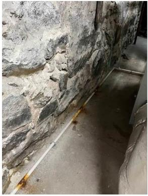
Sanitary line (leaking) in basement Mechanical Room
