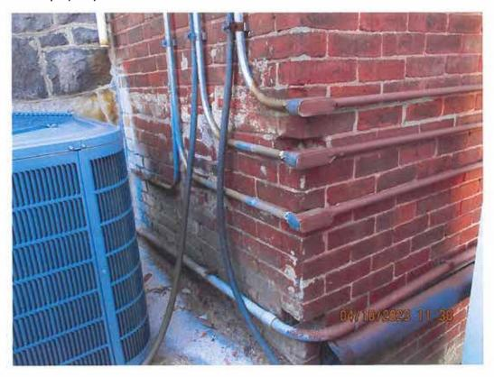
Chimney base in good condition except where brick was chiseled out for conduit bends
