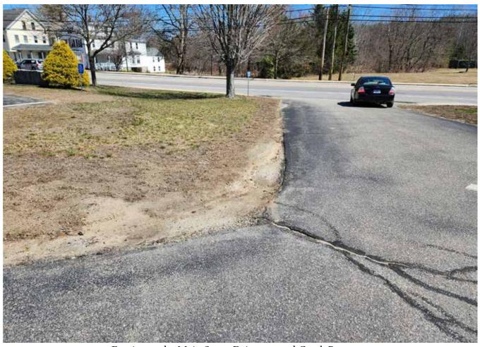
Erosion at the Main Street Driveway and Crack Pavement
