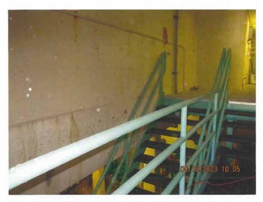
Masonry block walls on poured in place concrete beam
