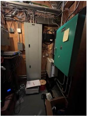
Main Distribution Panelboard on 2<sup>nd</sup> floor and defunct automatic transfer switch from previous, smaller generator
