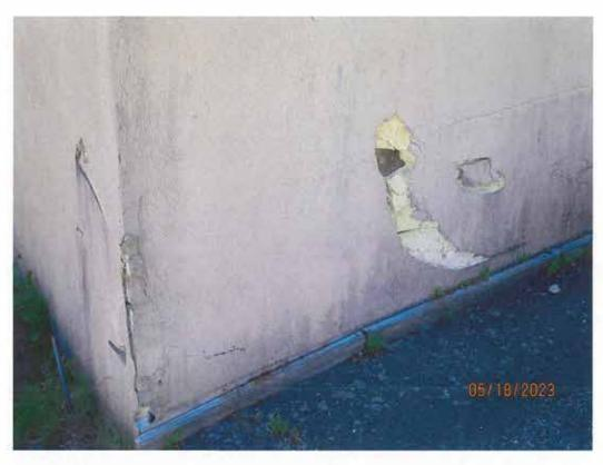
Damage to EIFS in the form of punctures, cracks, wear, & tear
