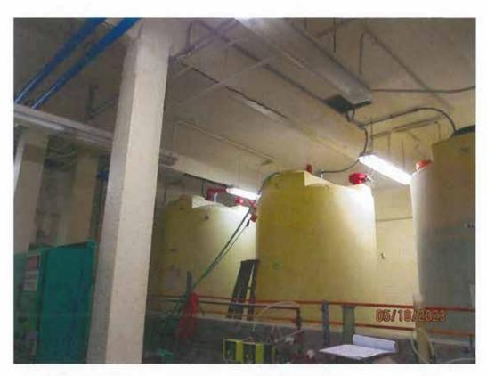
Chemical storage room, steel corrosion causing coating to fail
