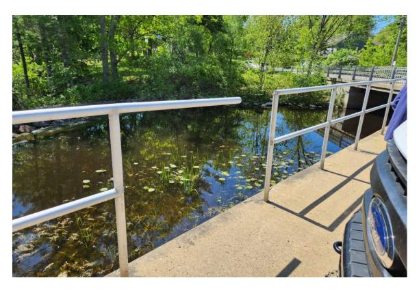
Handrail is missing and there is no car guardrail.
