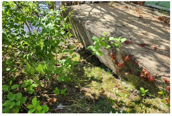
Erosion under slab out the rear of the building.
