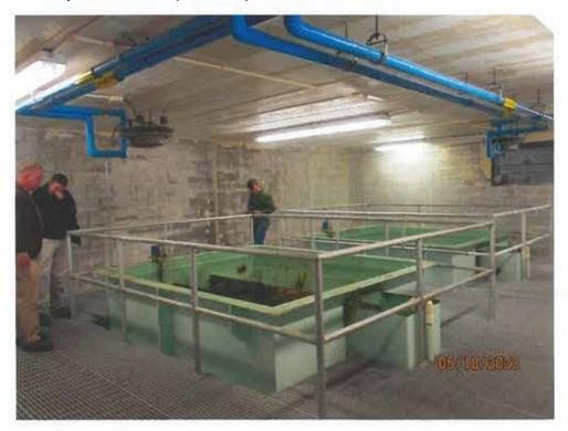
Pretreatment room with precast concrete roof panels
