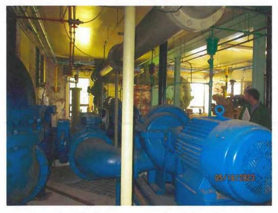
Pump room – steel framed floor supporting suspected wood floor joists
