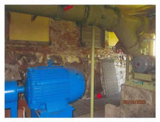
Basement pump room – original stone foundation wall & multi wythe brick wall
