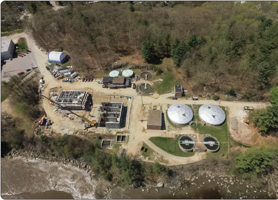
Wastewater Treatment Facility
