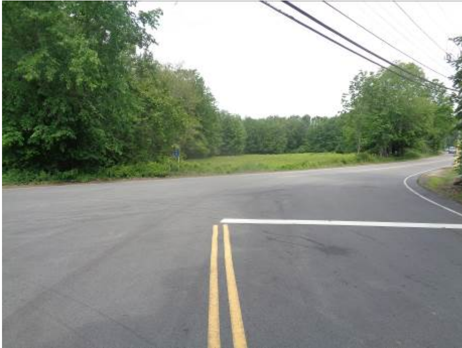
Front of the Subject Property – Front Upland Excess Area Looking Northeast from Grant Road - (6/23)
