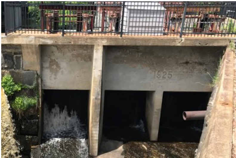
Leakage at gate structure
