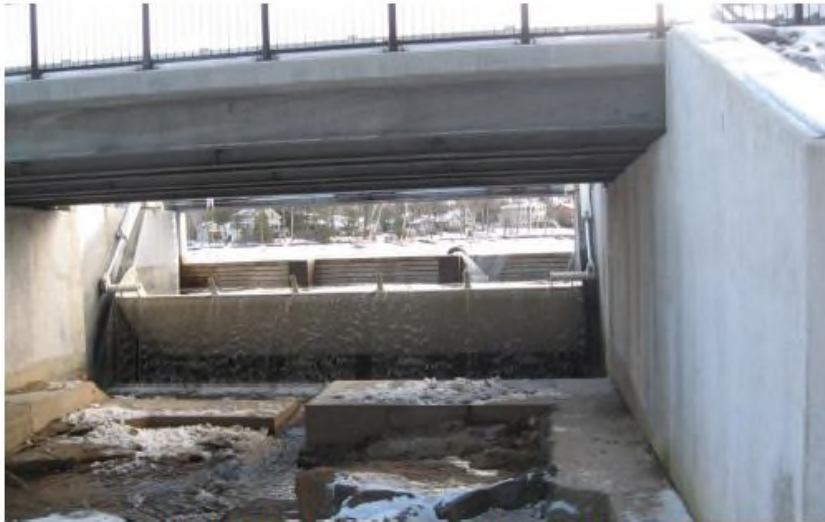
Hydraulically-Operated Crest Gate system. Otis Reservoir Dam, Otis, MA Image Source: GZA Construction Observation
