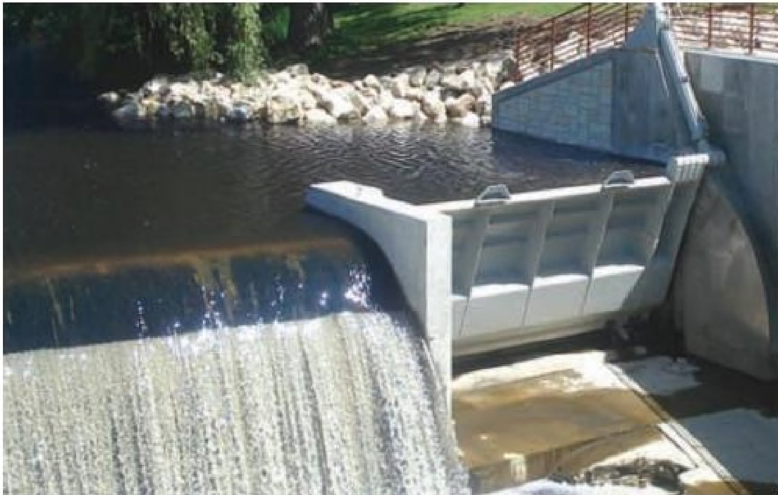
Hydraulically-Operated Crest Gate system.
