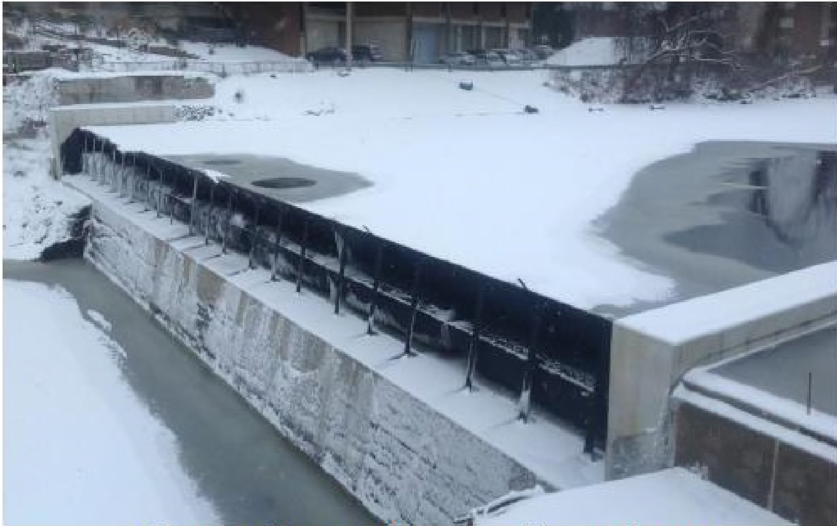
Obermeyer Spillway Gate system. Jackson Falls Dam, Nashua, NH
