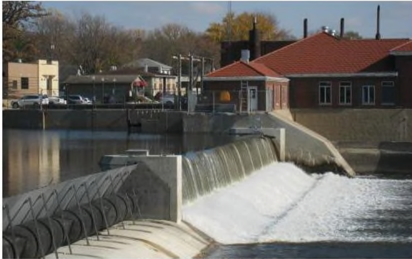
Obermeyer Spillway Gate system. Image Source: Obermeyer hydro, Inc. website.
