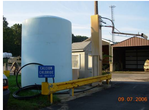
Figure 38. Overhead Pre-Wet Spray System
