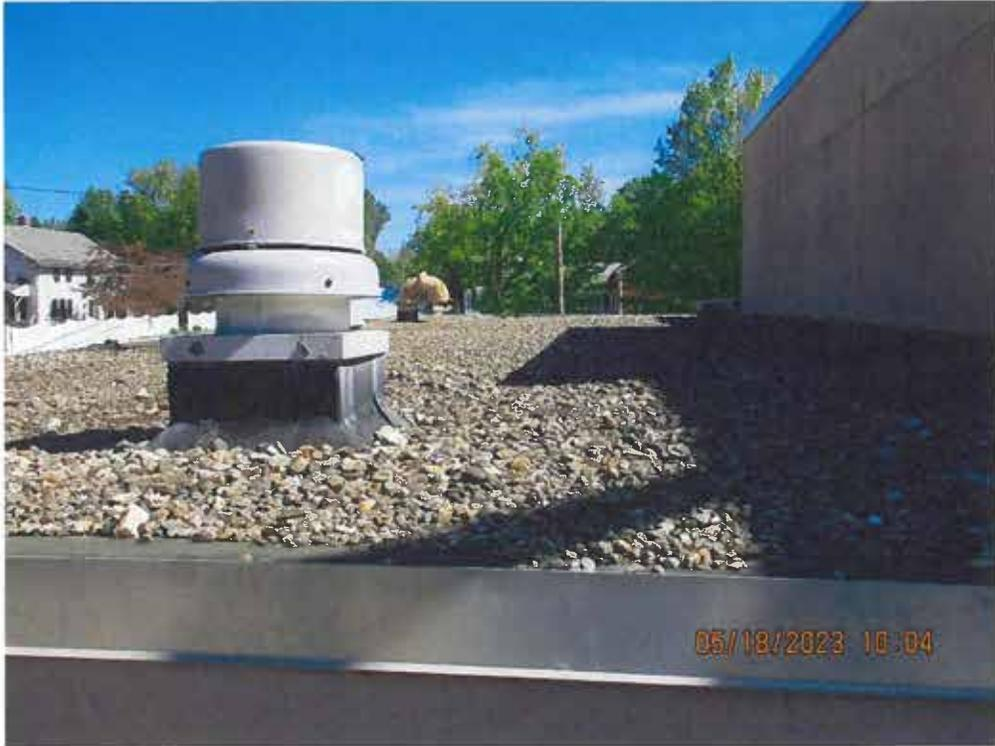
Membrane roof w/ ballast over chemical storage room
