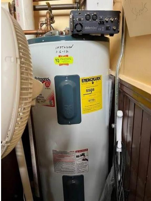
Electric tank-style water heater in IT/Storage Room in basement
