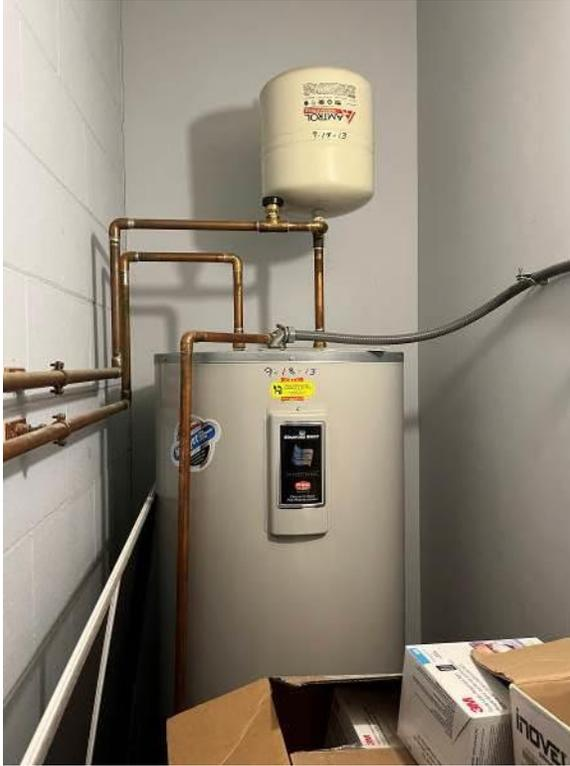
Electric tank-type water heater with expansion tank above
