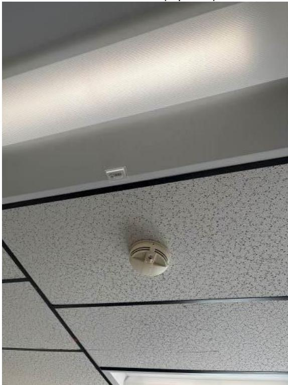
Line voltage smoke detector (not possible to determine whether these have any interconnection to the system fire alarm)
