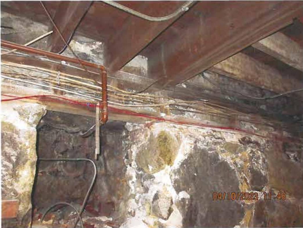
First floor wood floor framing rests on stone shelf. Wall framing continues to roof along with cut stone brick veneer.
