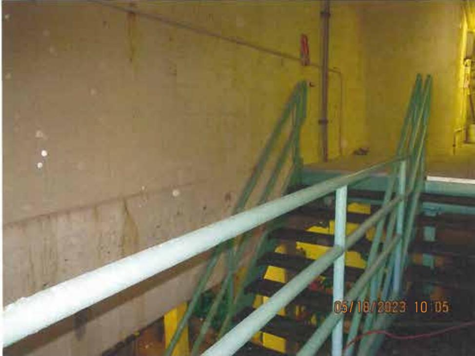
**Masonry block walls on poured in place concrete beam**
