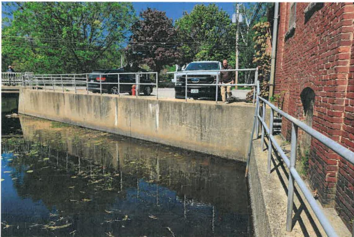
Integrated foundation/retaining wall/headwall/bridge abutment
