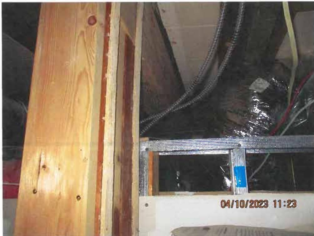
Tax Office 2 – Third floor reinforcing to allow opening in bearing wall on second floor
