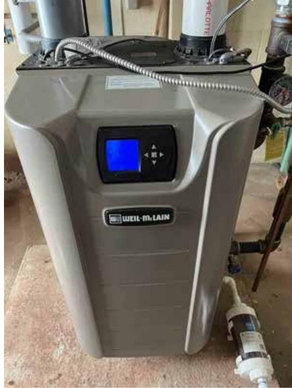
Gas-Fired Condensing Boiler
