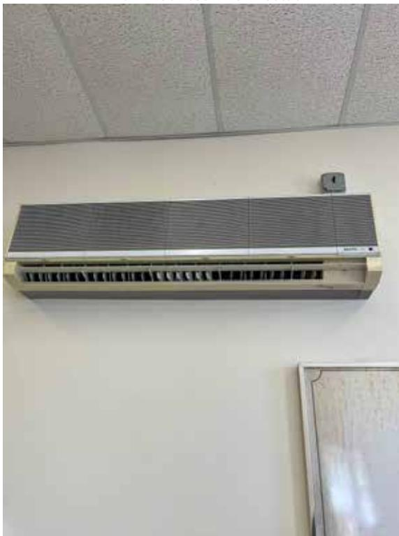
Wall Mounted Ductless Air Handling Unit
