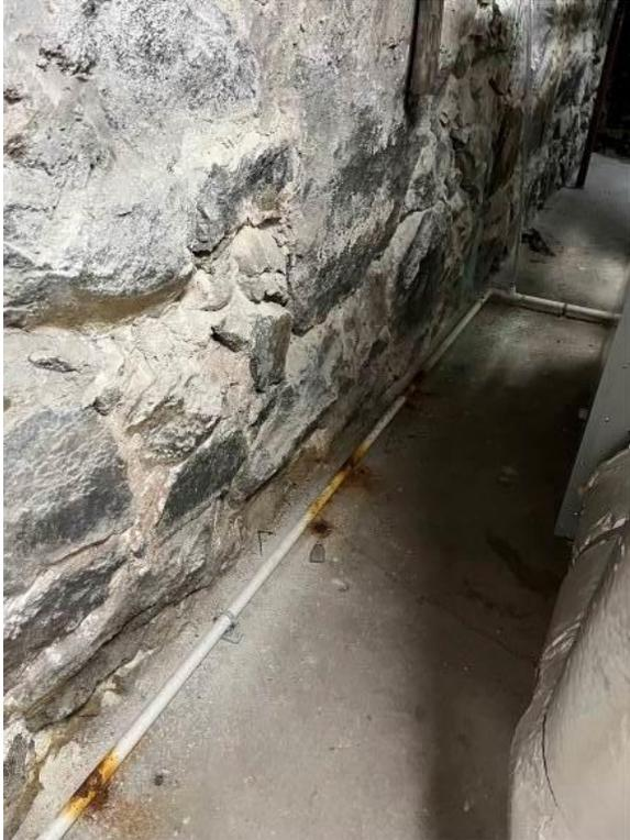
Sanitary line (leaking) in basement Mechanical Room
