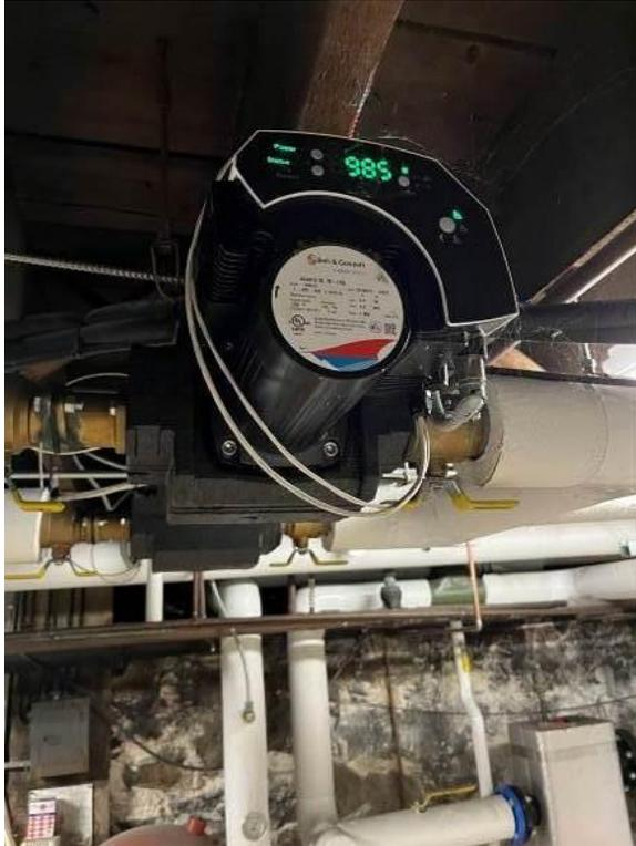
EC pump motor for hydronic heating system in basement Mechanical Room
