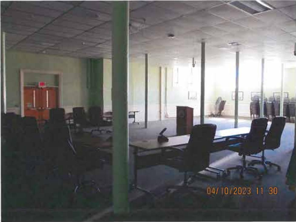
First level – posts align with above bearing walls
