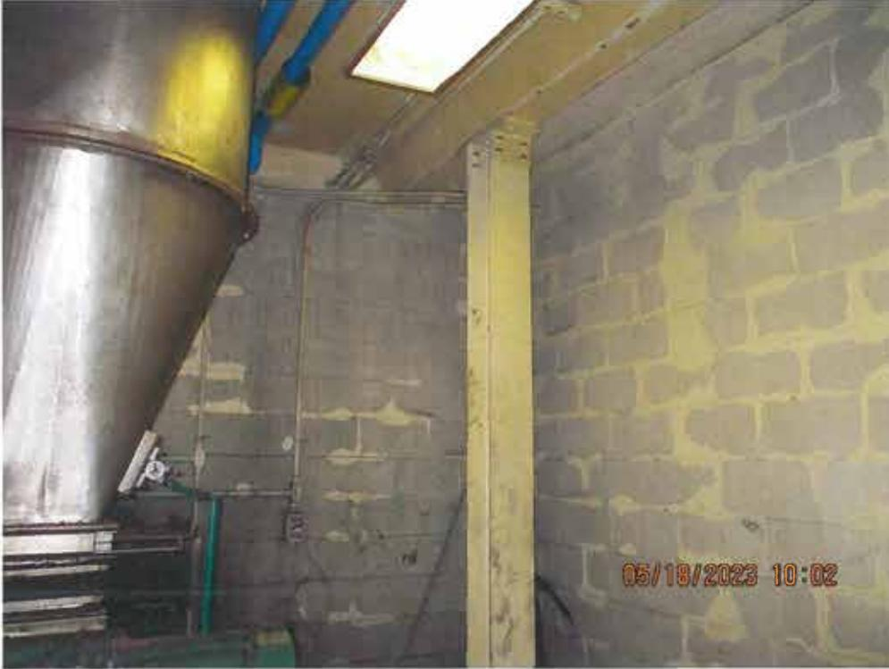
1990 Masonry block wall & steel framed floor
