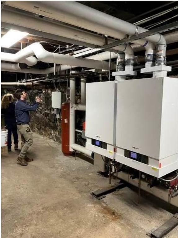
Condensing boilers in basement Mechanical Room
