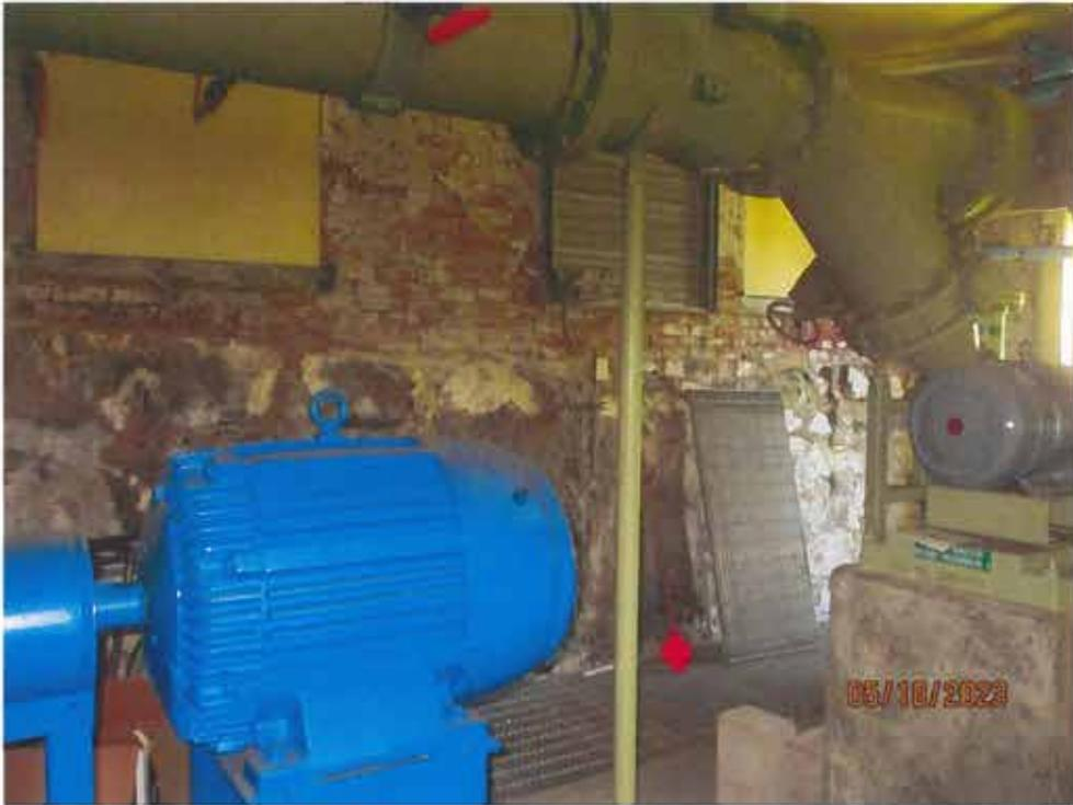
Basement pump room – original stone foundation wall & multi wythe brick wall
