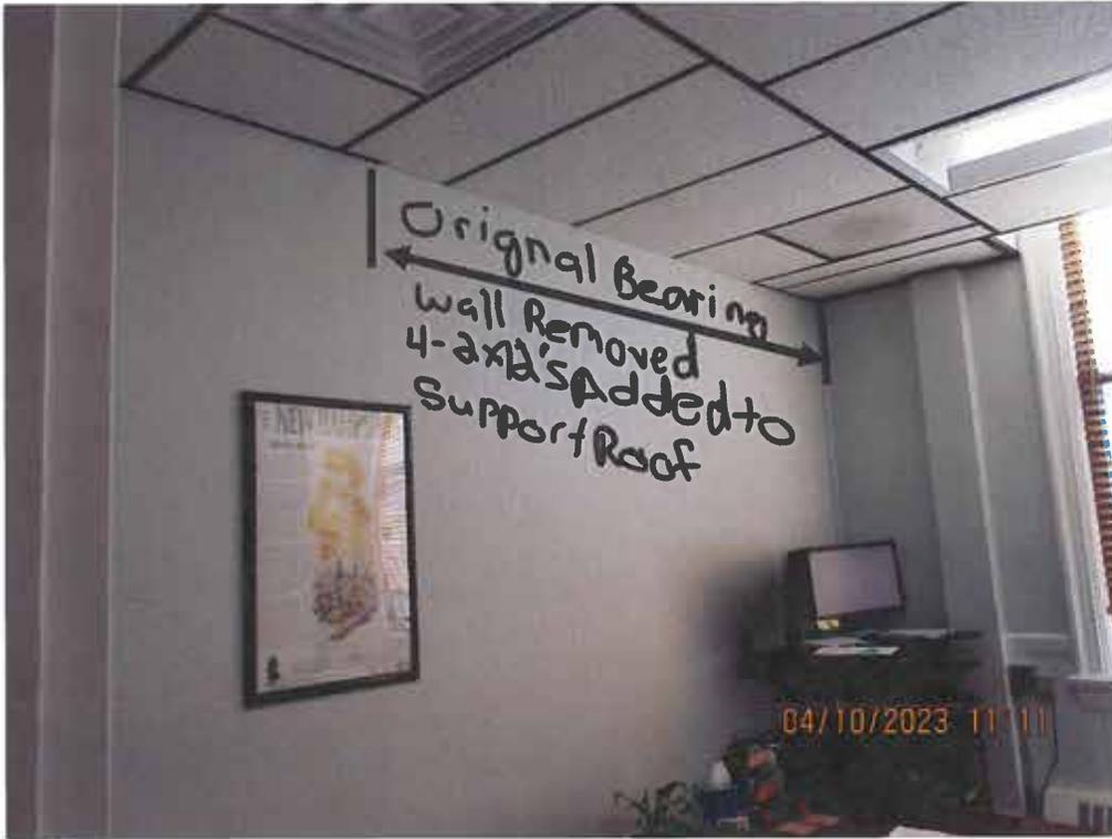
Third floor portion of bearing wall removed. New partition wall terminates at ceiling grid
