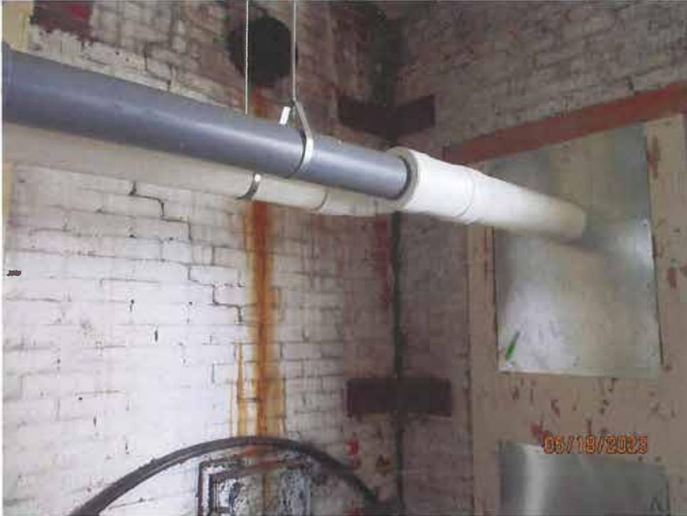
Rear wall exhibits crack at junction of chimney. Reinforced with stabilizing plates
