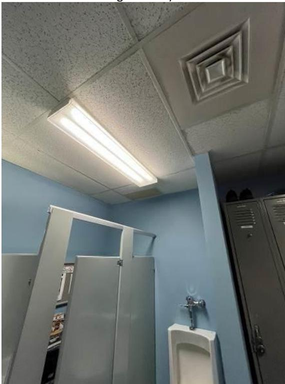
Bathroom with 4-way diffuser, fluorescent surface-mounted light fixture
