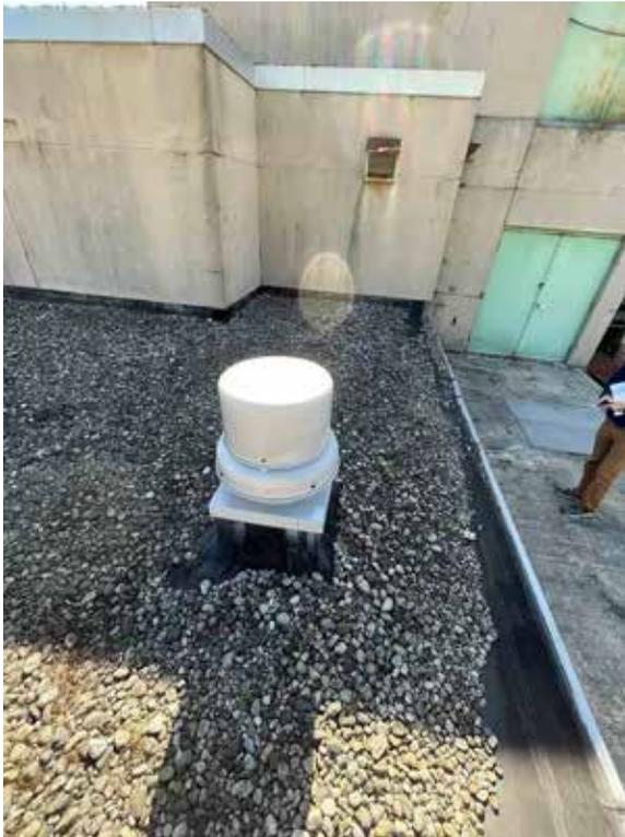
Roof Mounted Exhaust Fan
