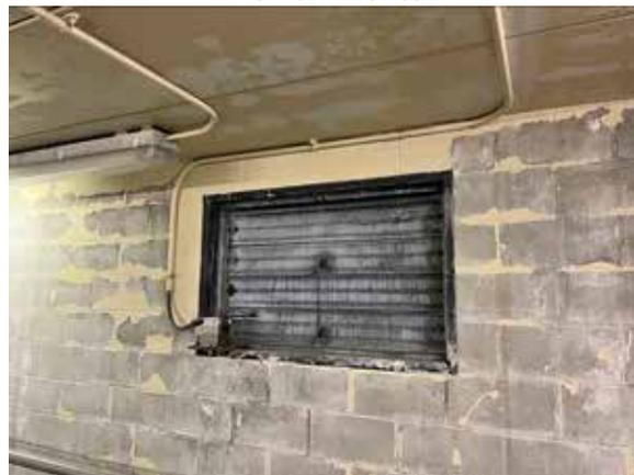
**Sidewall Intake Louver and Motorized Damper**
