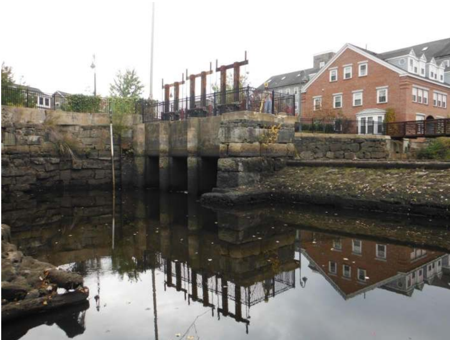
Figure 6:Left abutment and crest gates. Photo taken during the October 2013 drawdown.
