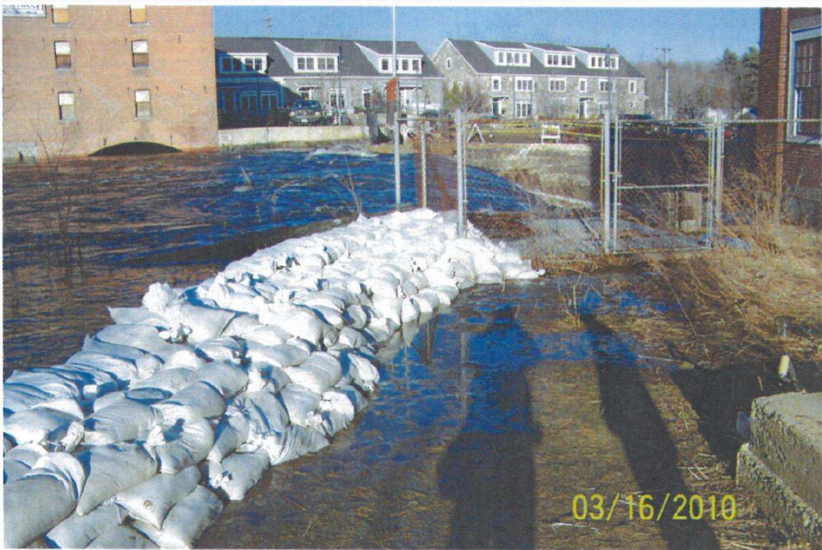
Figure 8: Macallen Dam during the March 16, 2010 flood event. Flow is approximately 6,710 cfs. Photo is taken from the right abutment, looking toward the spillway and left abutment. Photo source: NHDES Dam Bureau.
