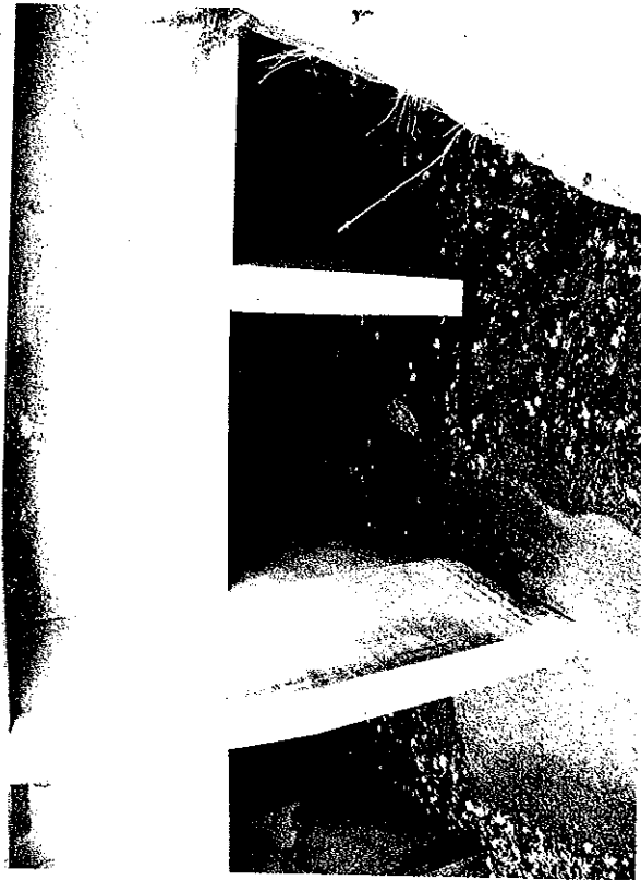
Leakage from low level gates
