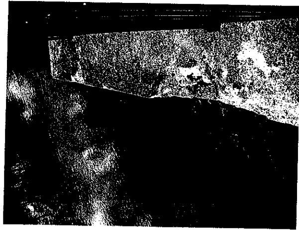
1. Concrete deterioration on upstream right abutment wall
