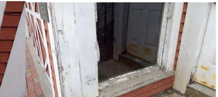
Window rot, glazing failure, sill rot
