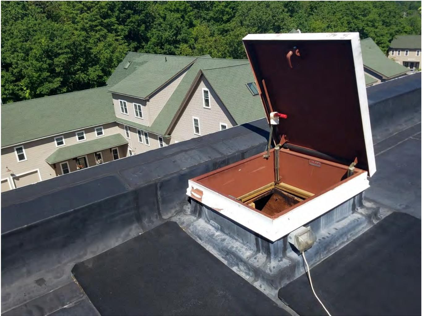
Town Hall Roof hatch No fall protection as required within 10 feet of the roof edge
