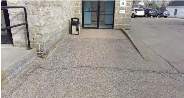
Town Hall parking lot repairs & Crack filling and seal coating
