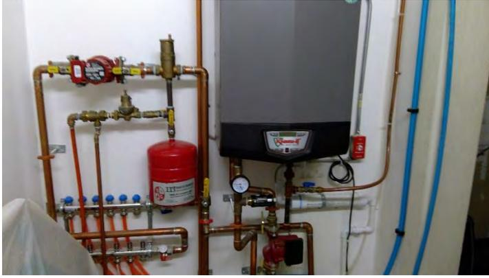
Radiant Boiler and piping (excellent condition)
