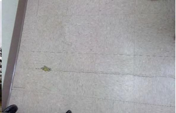
Slab separating and tile cracking
