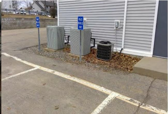
Condensing units (one unit new) (R-22 phase-out)
